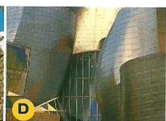
D Concrete, glass and metals are made from rock.
